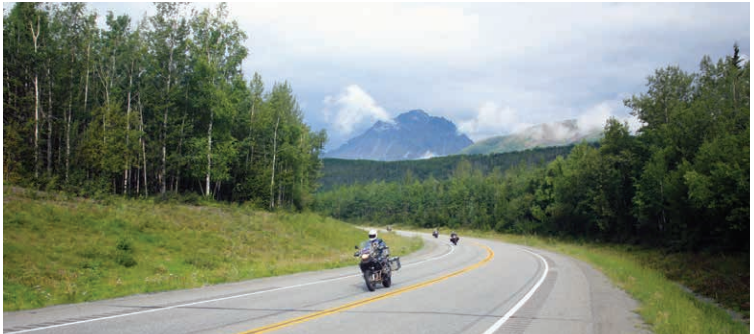
Palmer Highway, Alaska, USA
